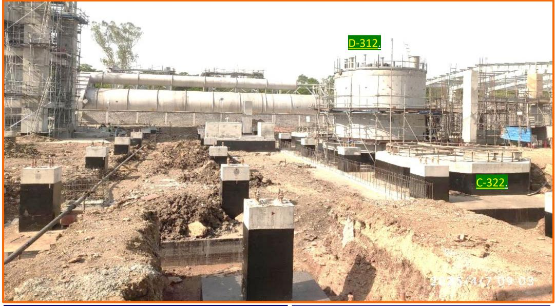
Raft & pedestal completed & backfilling work in progress. Trench RCC & Tank D-312 Erection work in progress.
